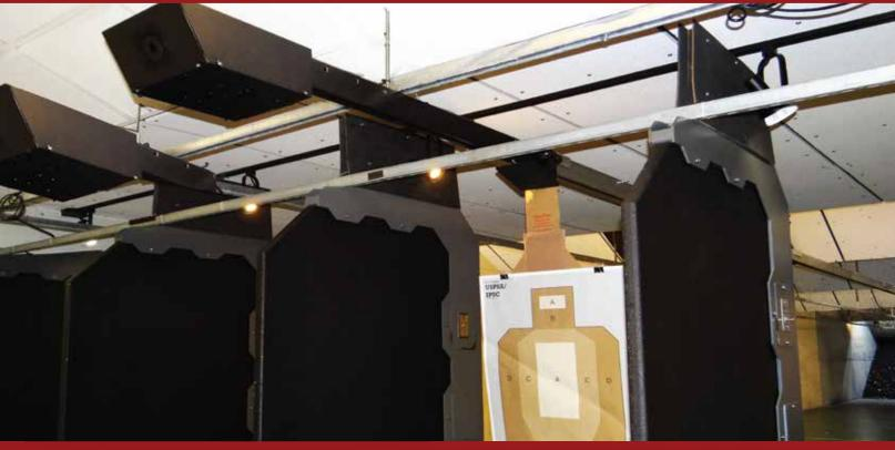
The Target Retrieval System (TRS) from SSI is critical for indoor shooting ranges. The TRS is a wire-guided static target on a motor-propelled carriage that smoothly travels along a suspended rail.
